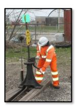
vii) Complete setting the switch by pushing down on the handle until it is fully inserted into the retaining notch. Insert lock or keeper.
